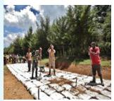
maintenance technique. "Do-nou" is a Japanese word that means wrapping soil in a gunny bag. CORE has operated in 27 countries worldwide since its establishment. CORE's main activity is spot improvement of community rural access roads utilizing locally available materials. So far, CORE has trained over 15,000 youths/farmers and repaired more than 165km of rural road. CORE carries out spot improvement of community rural access roads utilizing locally available materials.
