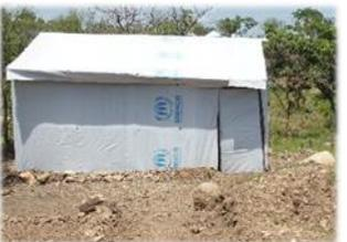
These shelters are feeble which causes leaking of rain. They also have a security problem since doors cannot be locked. In the next stage, materials are given and tools are lent to build a more durable houses. Refugees use mud bricks and mud mortar to put up walls, then thatch their roofs with wooden poles and dried grass. As a result of
